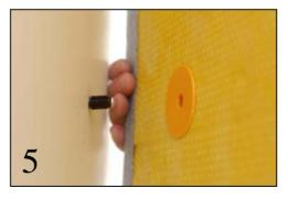
Firmly push panel onto ratchets to complete installation.
